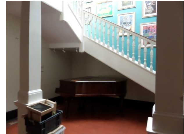
Ref: 2.2.3 Piano stored under Fire Escape staircase
