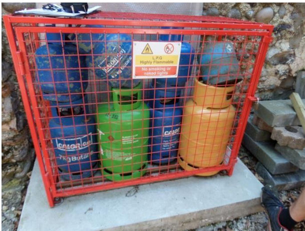
Ref: 1.2.3. Cylinders stored on top of each other
